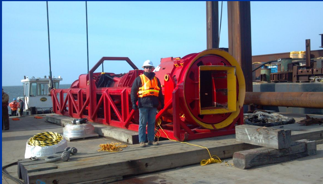
Pileco D225-22 for driving 36" Concrete Piles for Bonner Bridge
